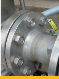
**To ensure** the optimum level of resources and verification is carried out on each joint, a criticality assessment will be carried out, which will consider the service, pressure and local conditions of each connection.
